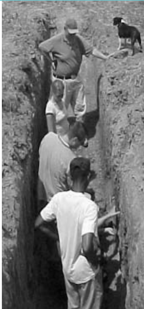
RCAP Technical Assistance Provider Richard Wise (foreground) works with the Indiana State Department of Health, the local department of health, and local residents to evaluate the soil at a proposed treatment site for on-site treatment or a package plant.
